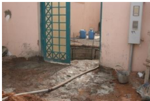
Picture (9) lack of maintenance
