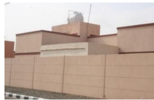
Picture (8) sewage holes that could easily open
