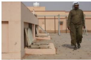
Picture (6) a well dug inside a house units front walls
