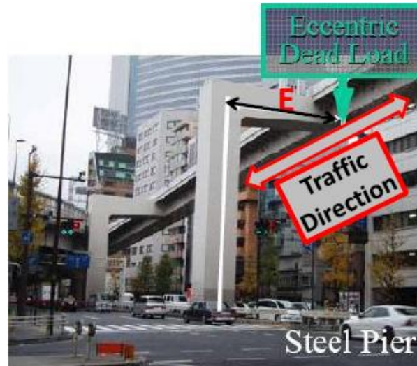
Fig. 2: Steel C-Bent Bridge Pier
