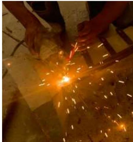
Figure 7: Welded Connections between Angels and Steel Stirrups
