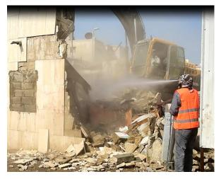
Figure 6. Water sprinkling in the demolition operation to reduce dust clouds effects [13]
