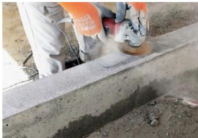
**Fig . 4:** Surface preparation by grinding
