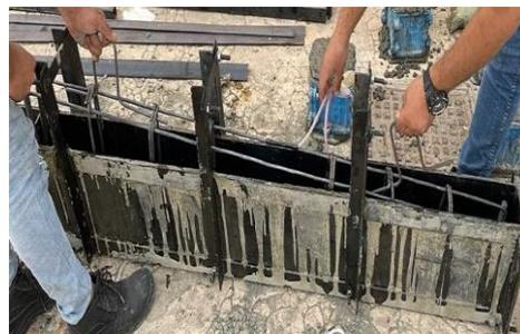
**Fig. 2:** The Specimens Before Concrete Pouring.
