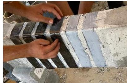
**Fig .5:**PlacingCFRP over the beam.
