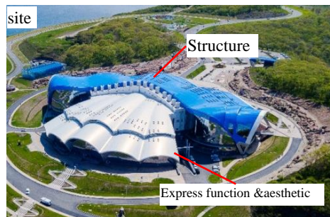
Fig. 3: Factors affecting the formation of aquarium museum Primorsky Aquarium Russia -Arch Daily.com [6]
