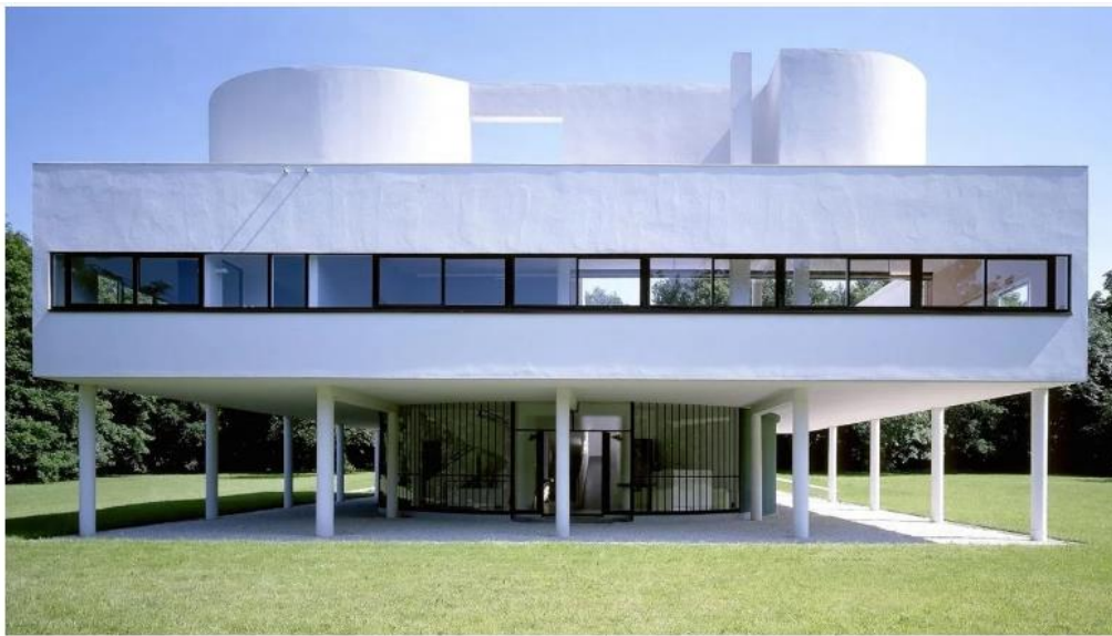
Fig. 3: House: Villa Savoye, 1931, Architect: Le Corbusier Style: Modernist
