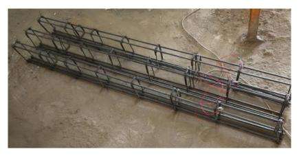
Fig.6. Reinforcement beams details.
