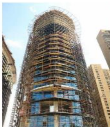
Fig. 6: Hotel towers in Cairo Maadi under construction Source: Researcher
