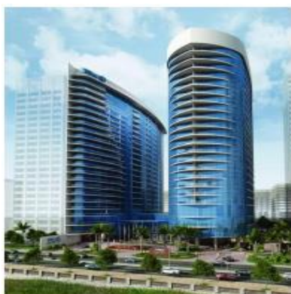
Fig. 5: Hotel towers in Cairo Maadi Source: Researcher
