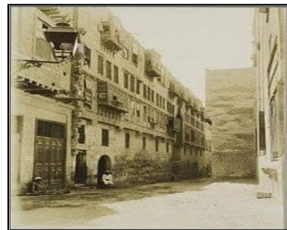
Fig. 20 The main façade before renovation
