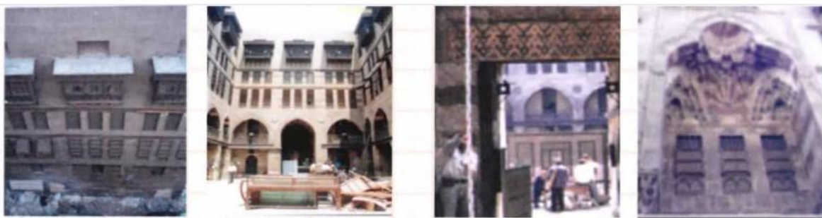
Fig. 21 The entrance facade overlooking the courtyard shows the poor condition of the windows and mashrabiyas due to weather factors, lack of maintenance, and accumulation of debris before the renovation process in 1990
