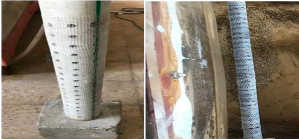
Photo. 3. Perforated Pipes and Gravel Filter For Wells.
