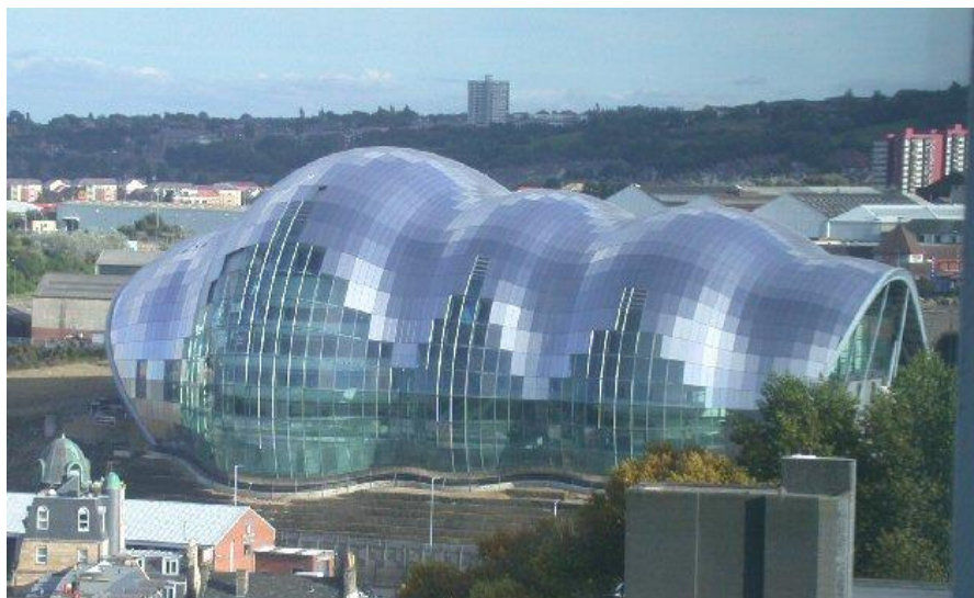
Figure (3): Bulge Architecture Pattern, Sage Gateshead Building in Gateshead, England. Designed by Norman Foster [49].
