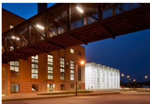
Fig.7. Construction of a pedestrian bridge among the building, the city, and the river[14]
