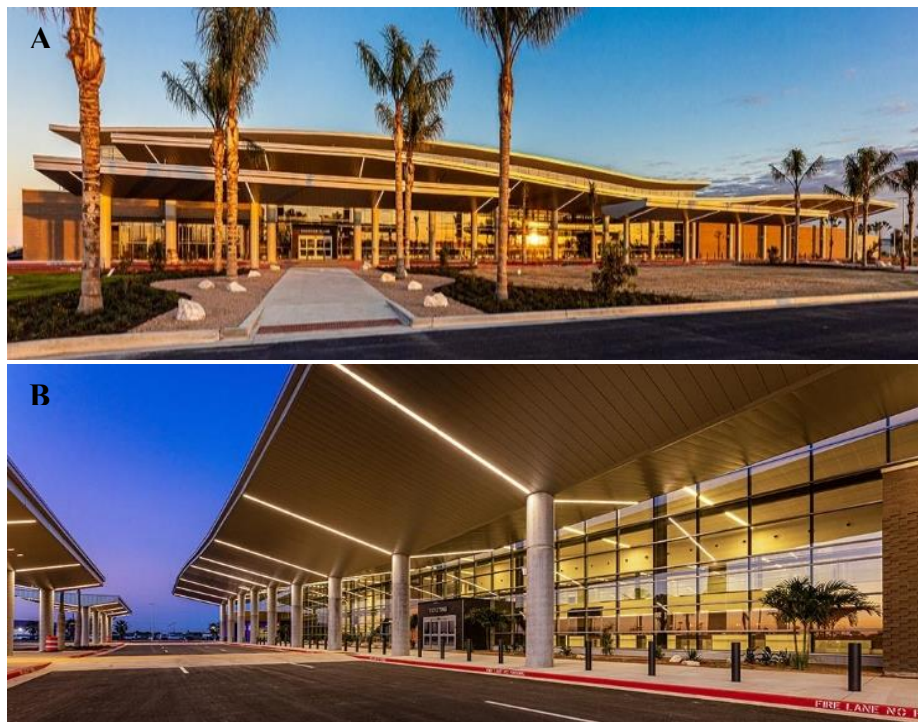
Fig. 26. Brownsville South Padre Island Airport: (A) and (B) different perspectives for the airport [31].
