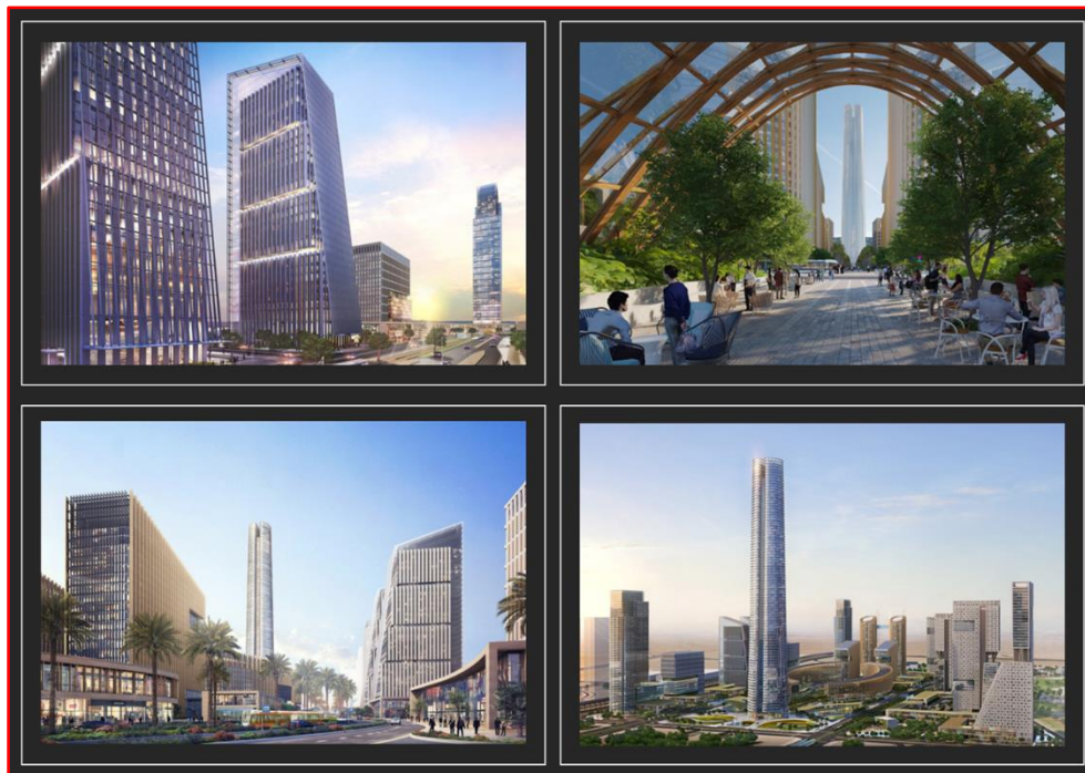
Fig. 7. Buildings in NACC [41].
