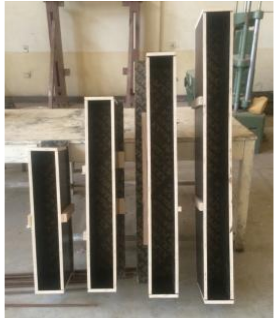
Figure [4] Wooden forms for columns casting
