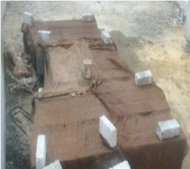
Figure [6] Columns curing
