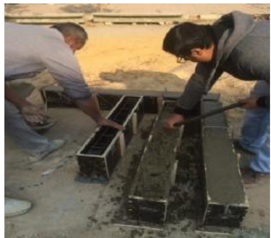
Figure [5] Columns casting
