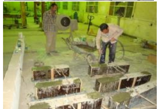
Figure [10] Replacement of damaged concrete by grout mortar
